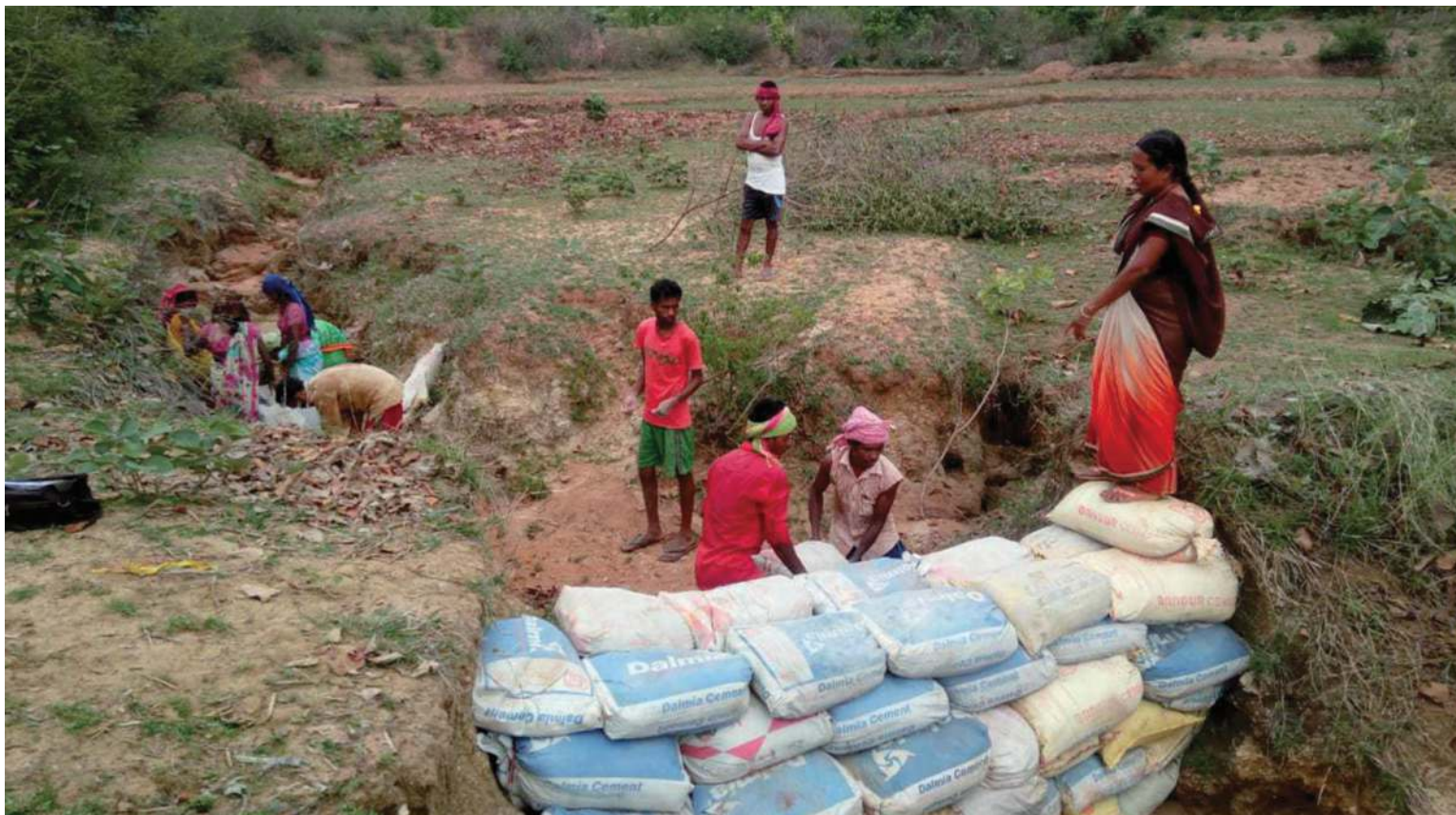
Chorha GP, Latehar, Jharkhand community builds a check dam
